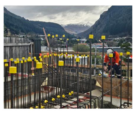
We continue to make good progress on the upgrade of the Queenstown zone substation, which supplies over 2,600 customers in the Queenstown and Glenorchy communities. The construction phase is currently underway, and following this we will install new 11 kV switchgear and replace the electrical protection and control systems. This project is on track to be completed mid-2025.
