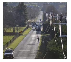
Customers in Momona, East Taieri, and Mosgiel are benefiting from upgrade work we have completed. We replaced 16 power poles, 72 cross arms, 4.2km of power lines, and seven pole-mounted transformers. Multiple crews worked together to minimise outage frequency and times as much as possible, in order to reduce the impact on customers and communities.
